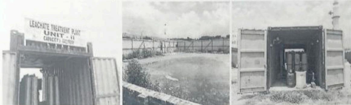
Figure 12: Existing Leachate Treatment Plant at Achan Site
