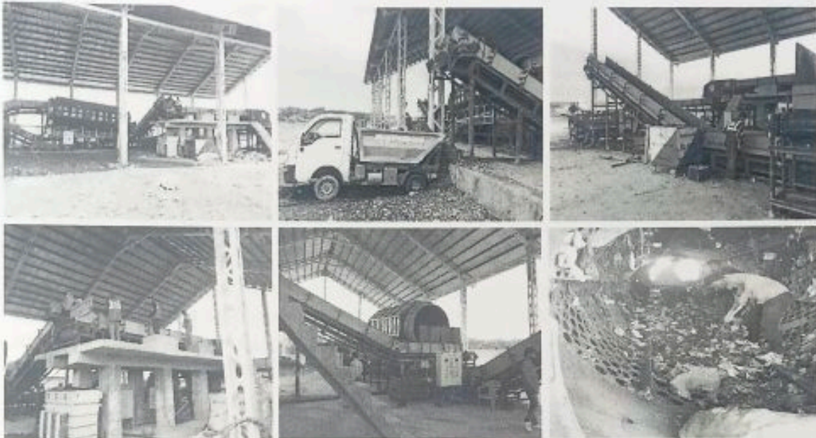
Figure 10: Mechanical Segregator & Compost Plant at Achan Dumping Site
